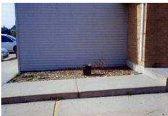
Before -- Front south side of the VFW Hall (note the bucket)
